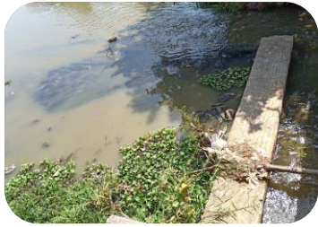
Uncontrolled sewage entry
