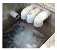
Backwash flow into feeding tank
