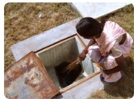
Removal of obstacle from the sewer pipeline
