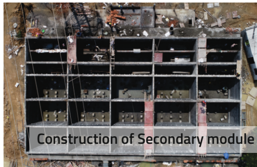
Sedimentation tank under construction
