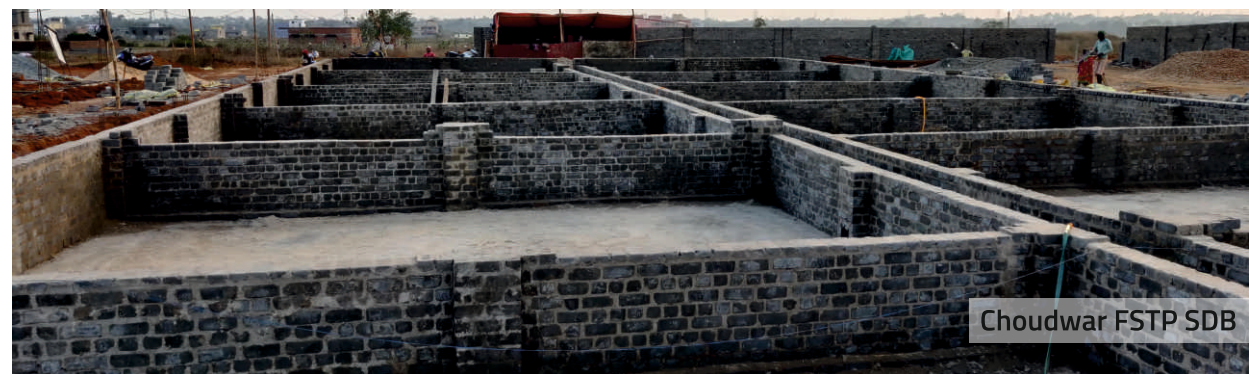
Figure 3 : Unplanted Drying Bed
