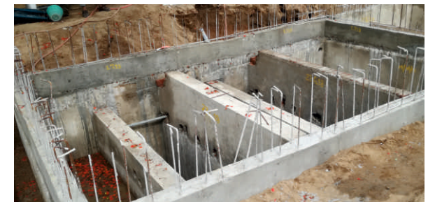
Figure 7 : Integrated Settler and Anaerobic filter
