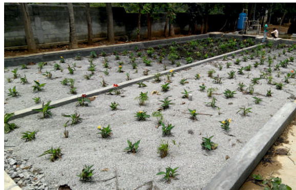
Figure 8 : Planted Gravel Filter
