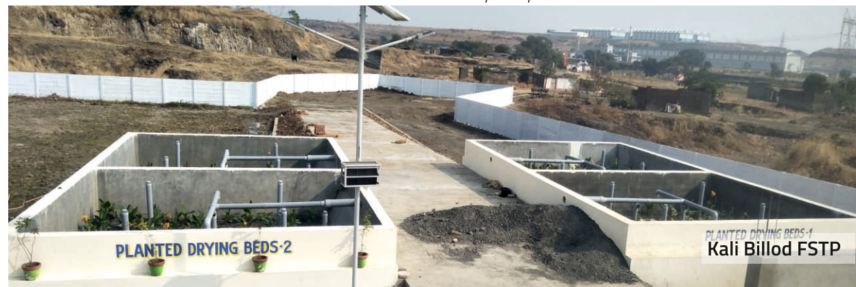
Figure 4 : Planted Drying Bed
