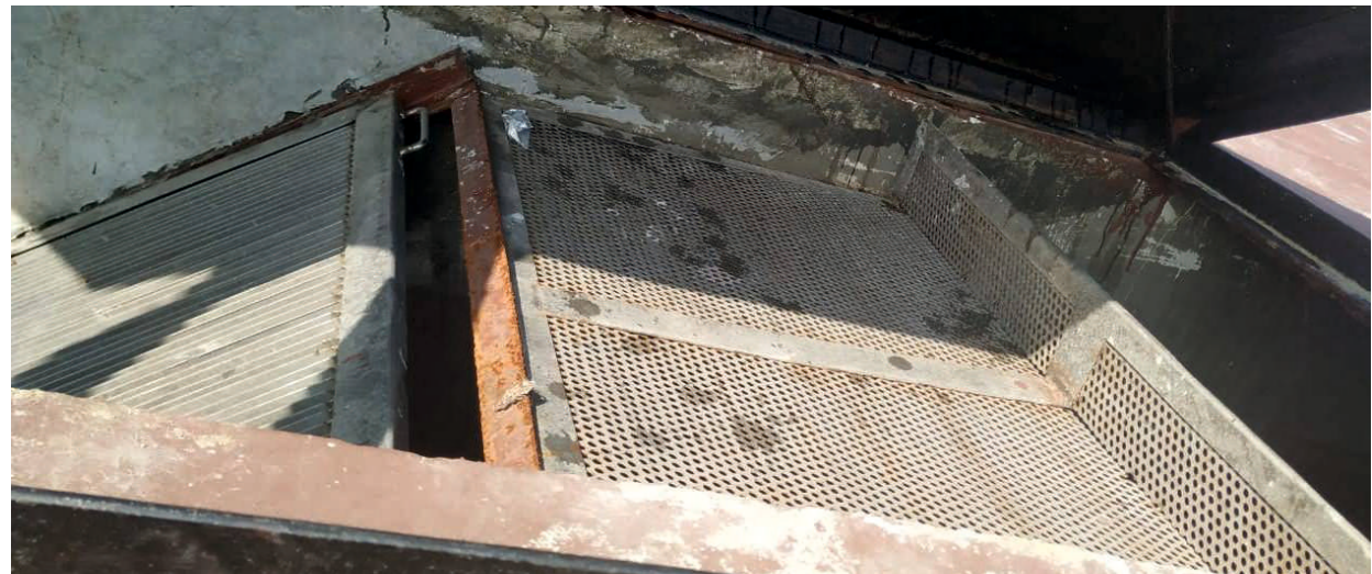
Figure 1 : Screen and Grit Chamber
