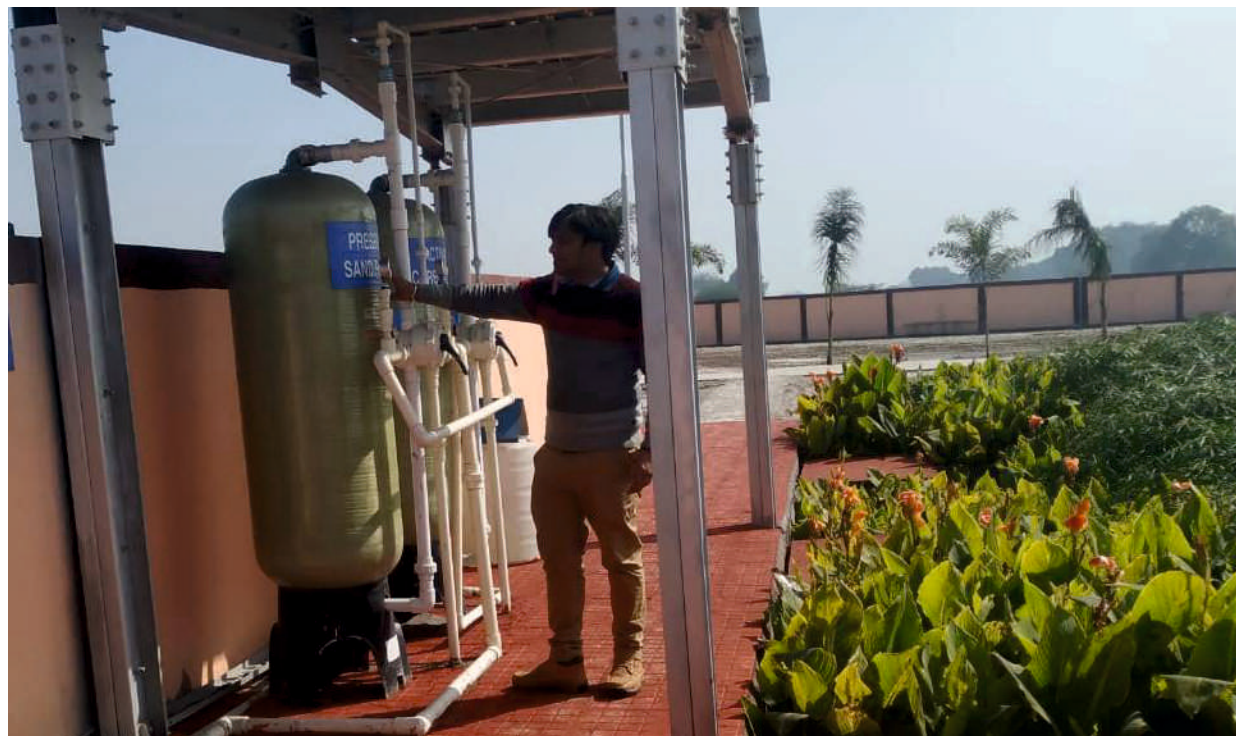
Figure 11: Final treatment of wastewater with Sand and Carbon Filter along with UV radiation method
