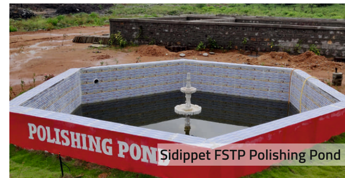
Figure 9 : Polishing Pond
