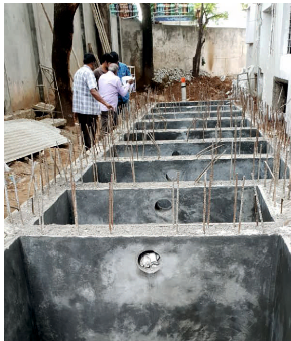
Figure 7 : Integrated Settler and Anaerobic filter
