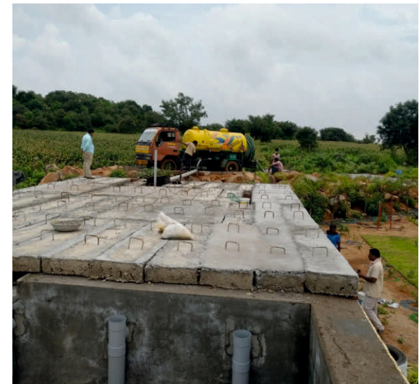
Figure 2 : Section of Sludge Stabilisation Reactor
