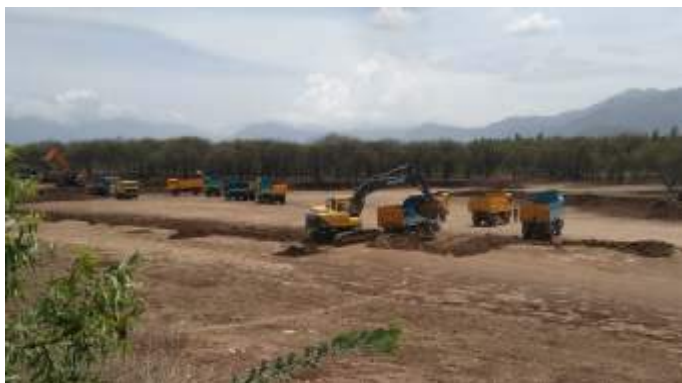
Desilting being carried out in Narasamapthy Lake during dry period
