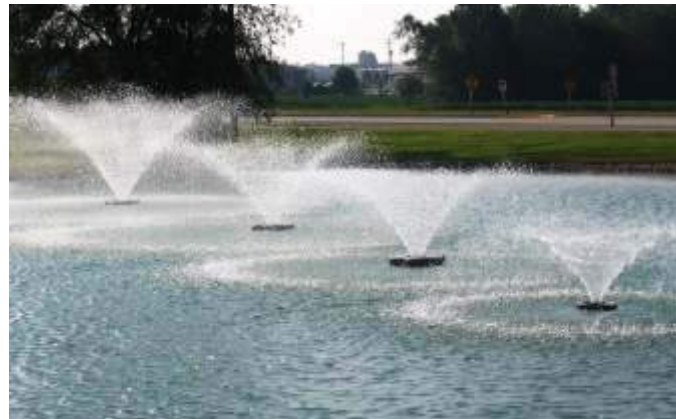
Surface Aerators to improve dissolved oxygen levels in the waterbody Photo courtesy: Kasco Marine
