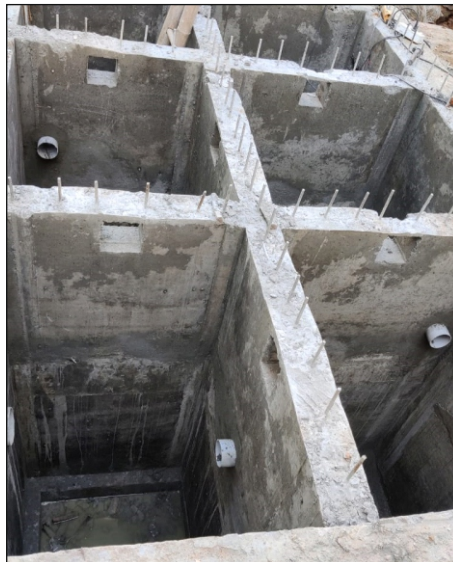
Completion of RCC wall construction
