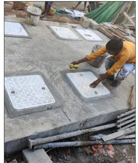
Fixing manhole covers
