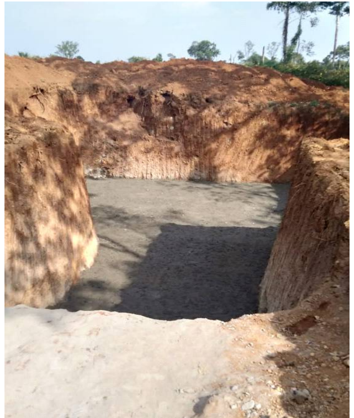
After excavation and finishing PCC (Plain cement concrete) work
