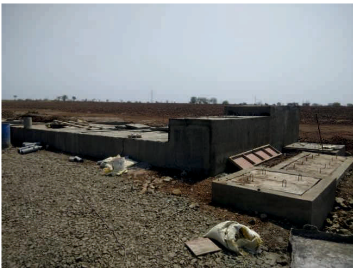
DEWATS during construction
