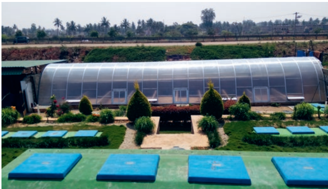
Photo: Mangalore tiles in a drying bed (top), sand added to the bed (middle), and greenhouses installed over drying beds (below).
