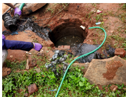
Solid waste in containment units blocking gulper operations
