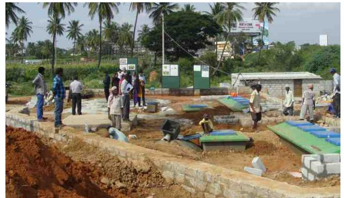
Construction site of the FSTP at Devanahalli. The plant can treat up to 6m<sup>3</sup> of sewage, of which the treated wastewater will be used for irrigation of nearby agricultural fields and the dried sludge co-composted with the municipal waste.
